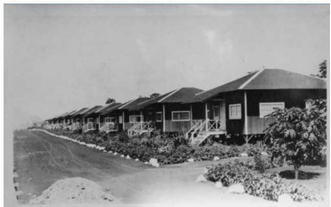
WACo worker housing, typical row, Hawaii State Archives
