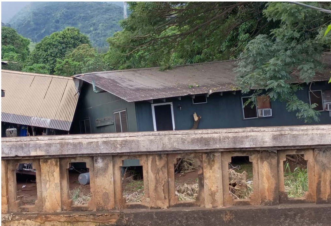
March 2026 - Kona Low Storms, Otake Camp house destroyed in the Waialua Floods. Photo O. Seyler
