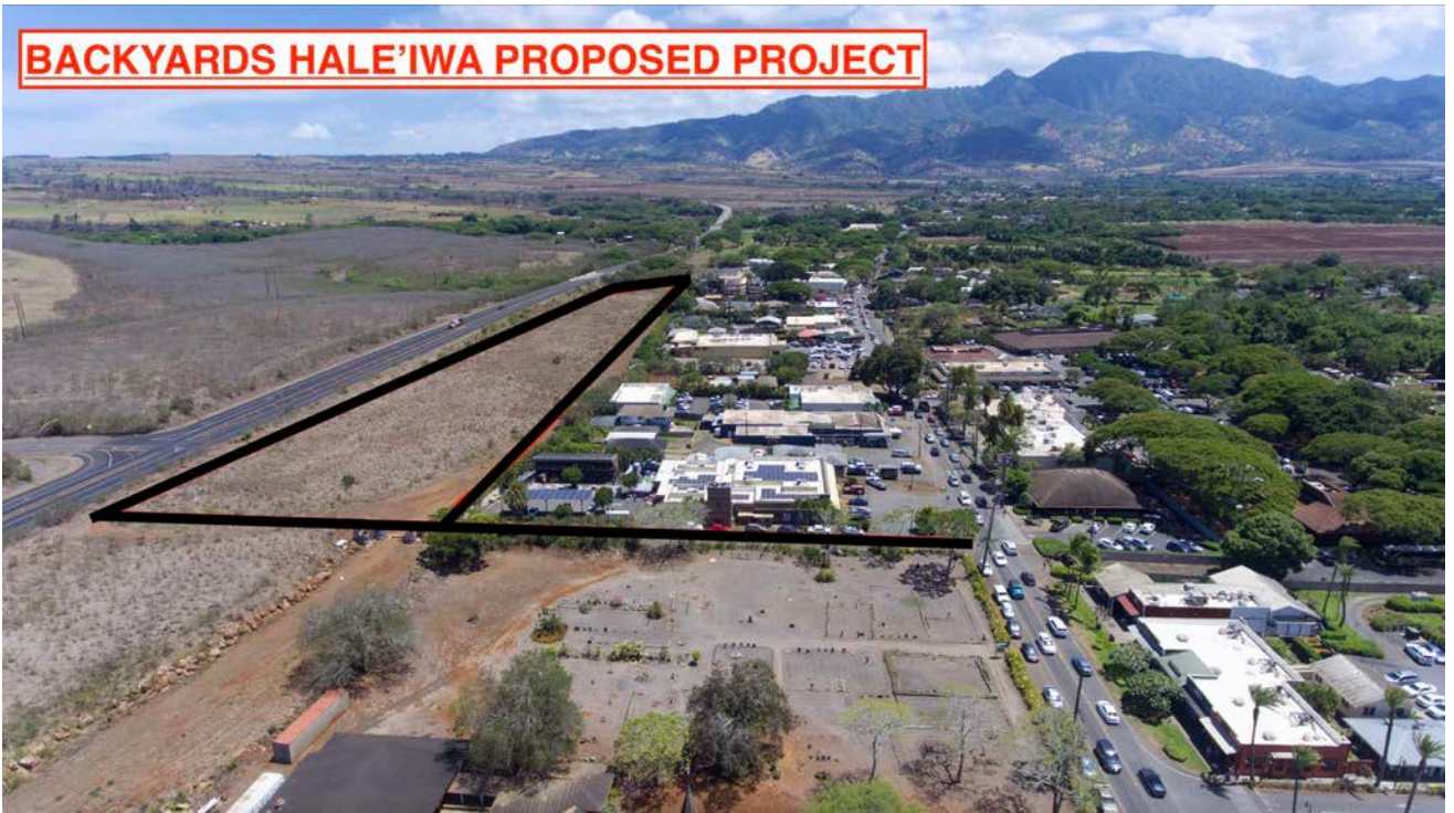
Hale'iwa Backyards Drone Shot: Zaz
